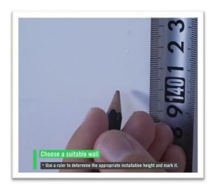
8. Punch position, the lowest part is at 140 cm, and then mark two holes (one is under the installer's left hand)
