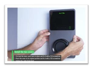
9. Tighten the AC cable fixing head
