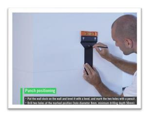
9. Drill two holes at the marked position (hole diameter 8mm, >50mm depth)
